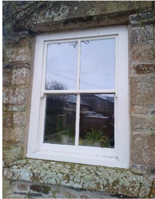
Double glazing in these examples at a farmhouse near Venterdon have been installed within original windows and frames.
