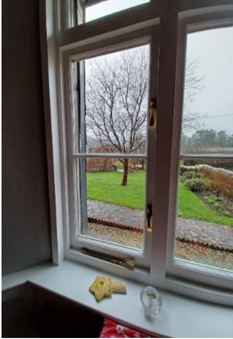
Double glazing in these examples at a farmhouse near Venterdon have been installed within original windows and frames.
