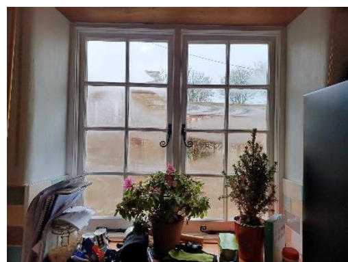
Double glazed replica windows at this farmhouse near Lockett on the left have glazing bars much thicker than the slim glazing bars of the remaining original windows in the same house on the right.
