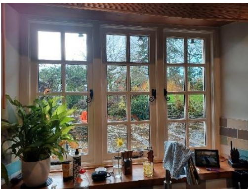
Double glazed replica windows at this farmhouse near Lockett on the left have glazing bars much thicker than the slim glazing bars of the remaining original windows in the same house on the right.
